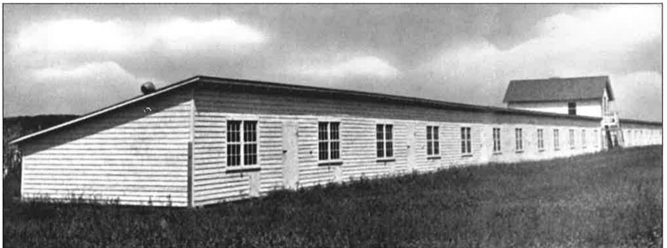
An example of the many long, narrow, shed-like broiler houses constructed in the 1930s and 1940s. Note the chicken house apartment on the second floor and the feed storage room on the first floor in the middle of this two-story chicken house.
