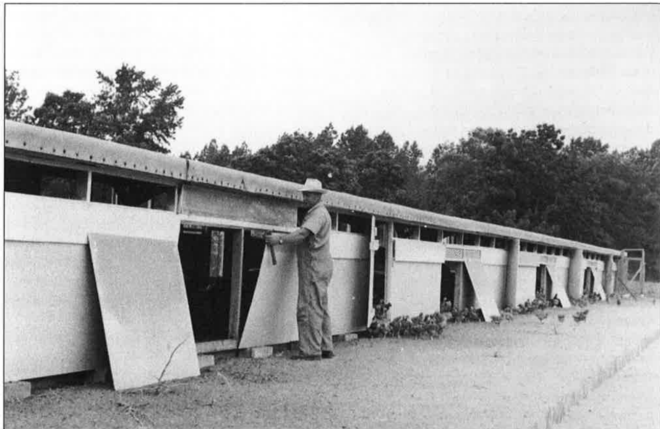
In the early 1950s, prior to the use of fans for ventilation, growers used a variety of ways to provide “natural ventilation.” Here large panels are being removed to allow greater air movement.
