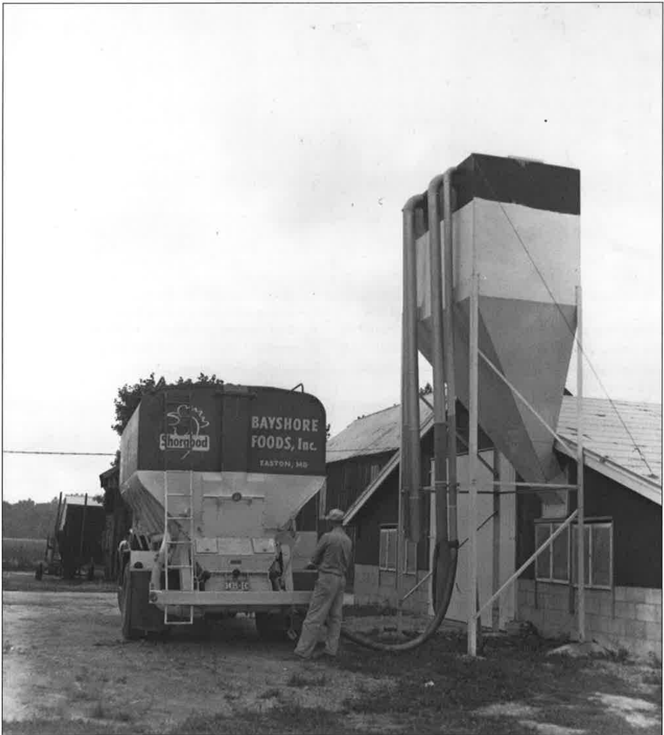
Early bulk feed handling with pneumatic truck and gravity flow bin in the 1960s.
