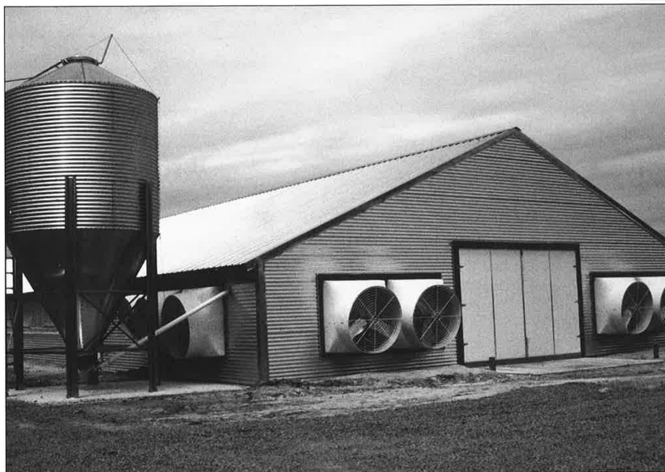
A chicken house of the 1990s. Many growers switched to tunnel ventilation of houses. As shown here, large fans on one end pull air through the entire length of the house. Though more expensive to operate than previous air movement systems, tunnel houses are designed to provide more uniform air movement and better living conditions for birds.
